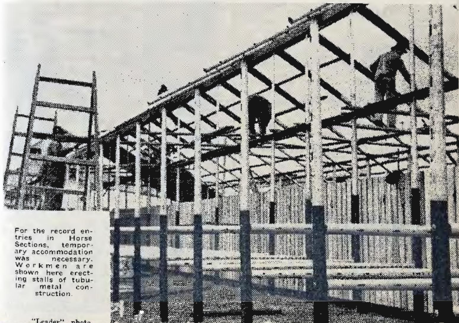
For the record entries in Horse Sections, temporary accommodation was necessary. Workmen are shown here erecting stalls of tubular metal construction.
