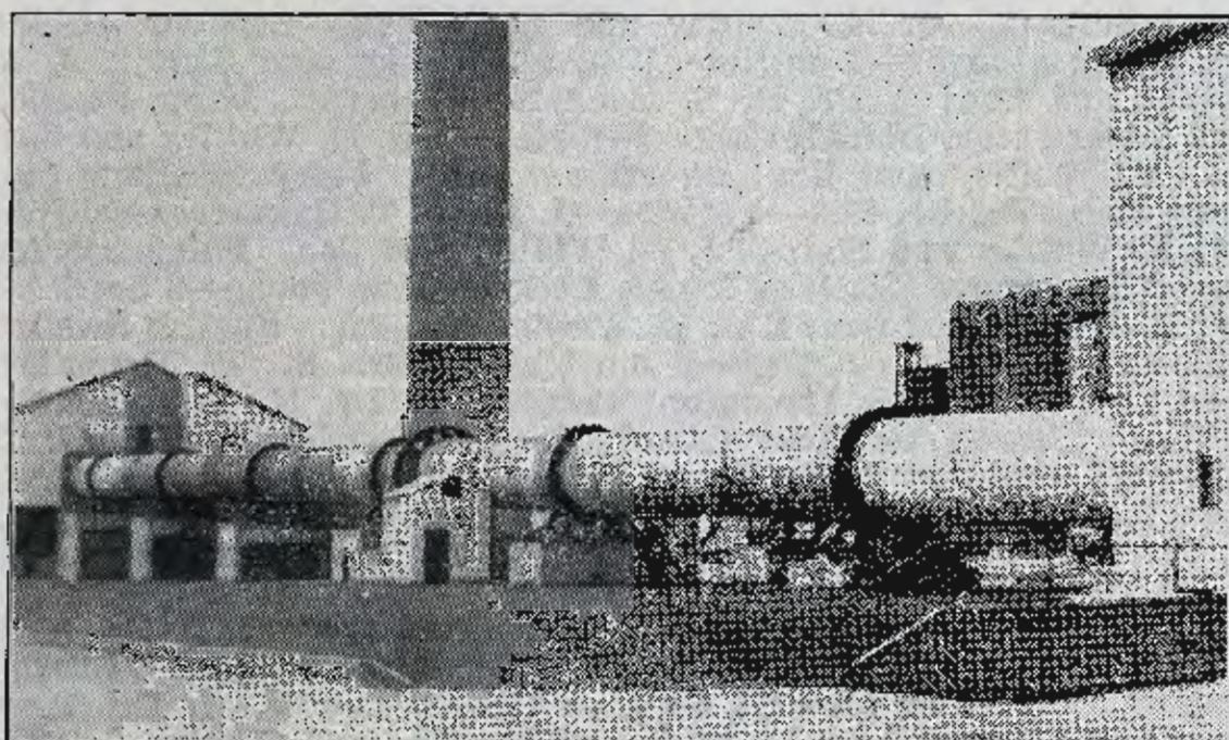
Large Rotary Kiln at Cement Works,
