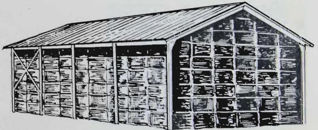
Portal Construction is no "pruned down to price" structure . . . it is absolutely top quality. ANDASTEEL portal farm buildings are fabricated from heavy channel with angle steel bracing and ties—all of at least 3/16" thickness. In storage you get far greater capacity than any other similar building because of the higher roof pitch and absence of internal members. Standard sizes are 60 ft. x 20, 25 or 30 ft. spans with 14 ft. wall height.
